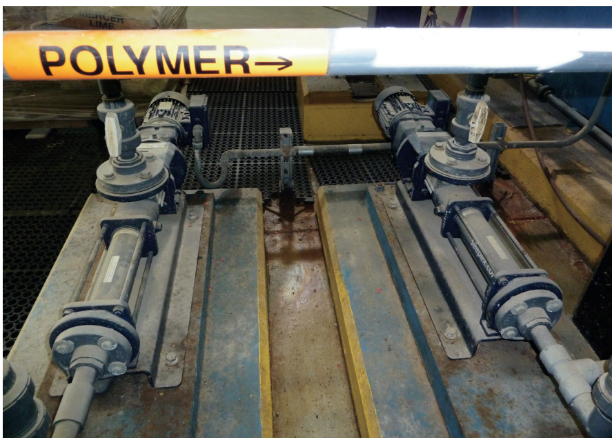
Progressive cavity pumps used to transport flocculants
