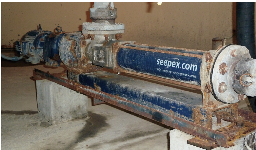
Right view of a PC pump that transfers the clarifier underflow or sludge to the dewatering system
